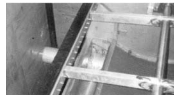
Self-cleaning trough for automatic screening
