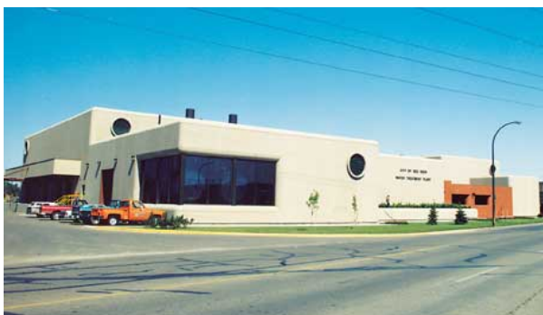
The Red Deer Water Treatment Plant
