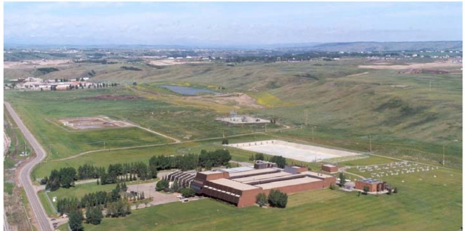
Bears paw Water Treatment Plant
