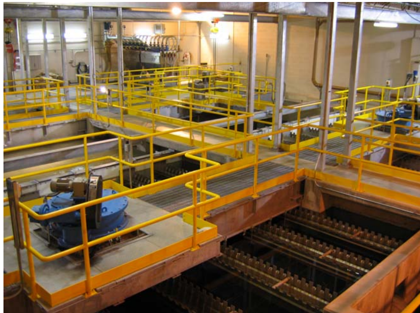
The ACTIFLO clarifiers were built inside one of the existing clarifiers
