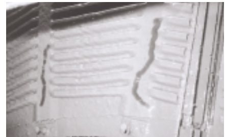
This is an example of the thinness of the fixed film biomass growth.
