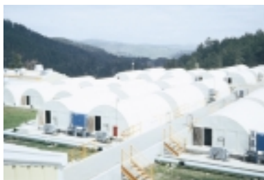
Process water used by one of the world's largest gold mines is treated by this USFilter RBC plant.
