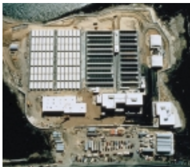
A major RBC installation is installed at a regional resort area near a major metropolitan city. Discharge is into an environmentally sensitive waterway.
